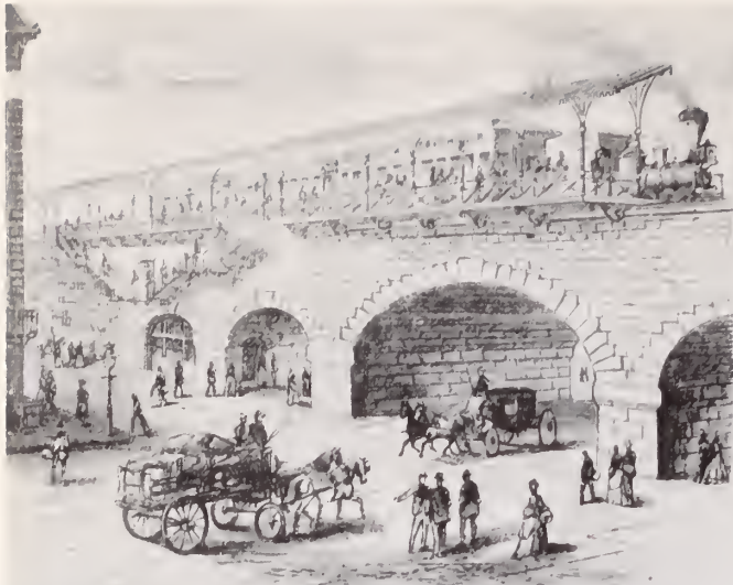
THE STONE VIADUCT FROM 99TH TO 115TH STREET—THE STATION AT 110TH STREET.
